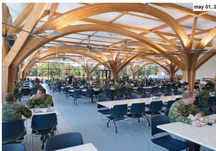
ZAS architects' Canadian military dining hall features tree-like columns made of glu-lam
